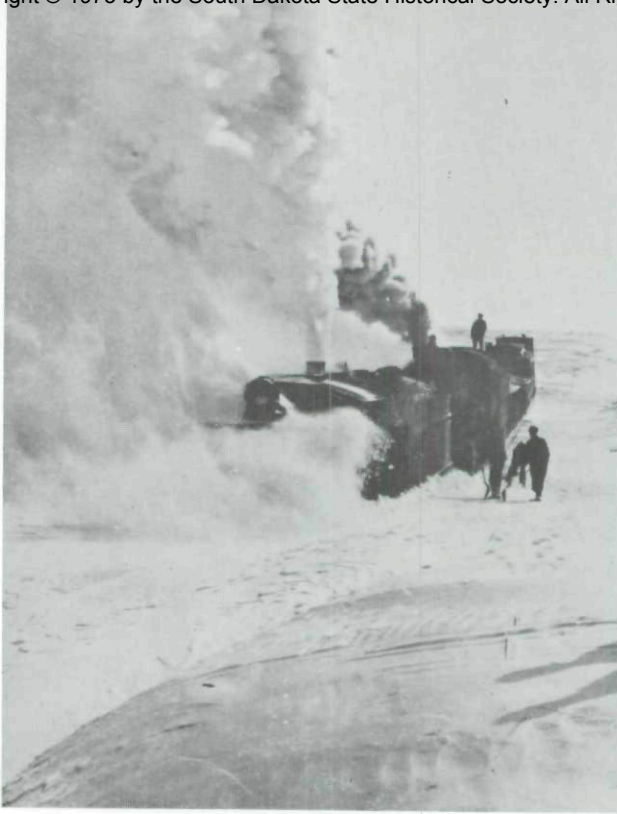
During the winter of 1922 a M&StL rotary plow was dispatched to clear the road near Conde.
