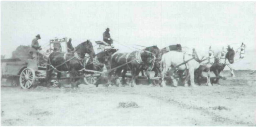
Horse teams pull an elevating grader along a new road bed in this view of a 1920s construction operation much like the one that fascinated Lingo.
