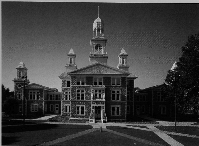
Constructed of pink quartzite, Old Main at the University of South Dakota in Vermillion was one of Wallace Dow's many commissions for college buildings. (Photograph by Scott Myers, Columbia, Mo.)
