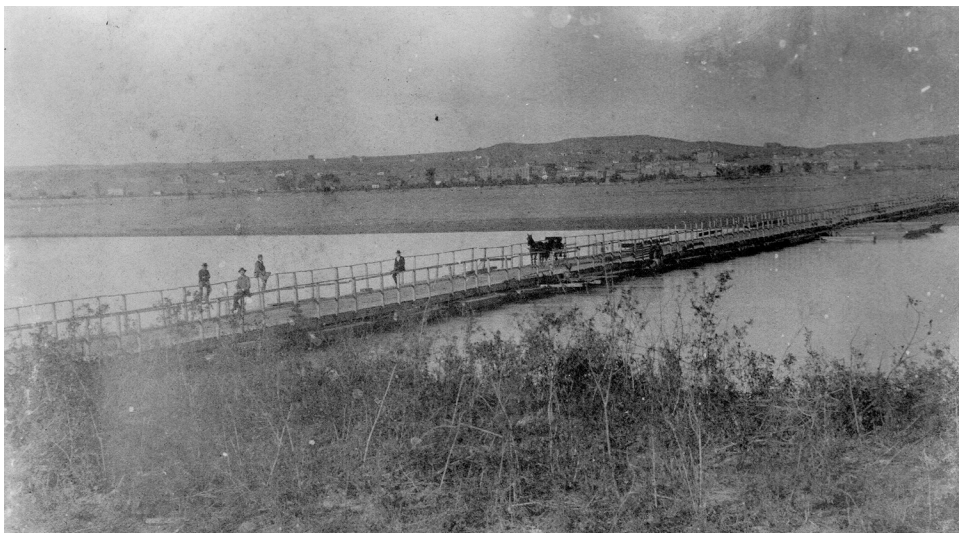
Pontoon bridges on the Missouri River provided a temporary but relatively cheap way to connect the towns of Pierre and Fort Pierre. This example was constructed about 1891.
