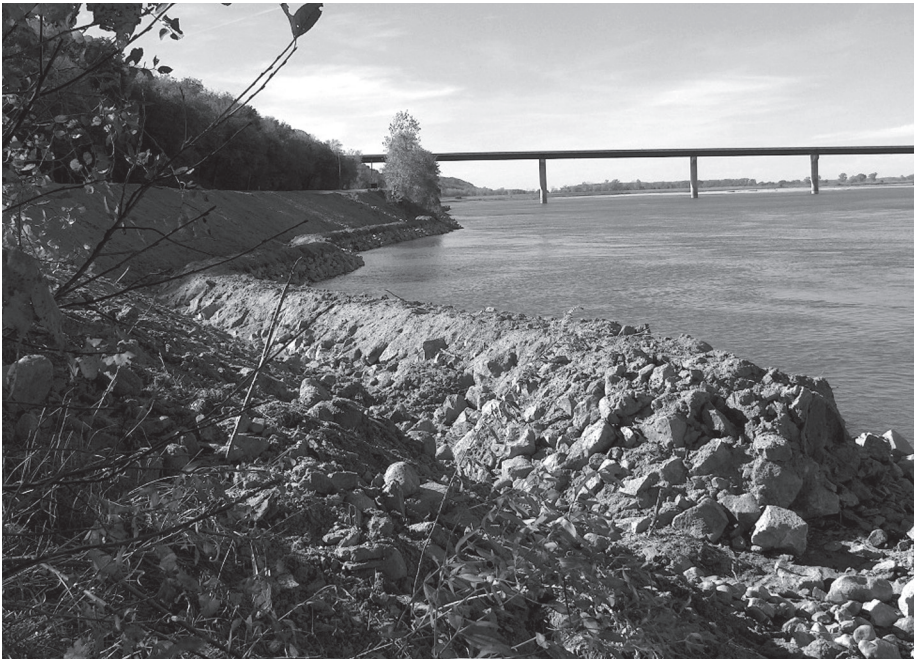
Rock lines the water's edge as part of a stabilization project completed in 2005 to protect a road in Nebraska's Dixon County.
