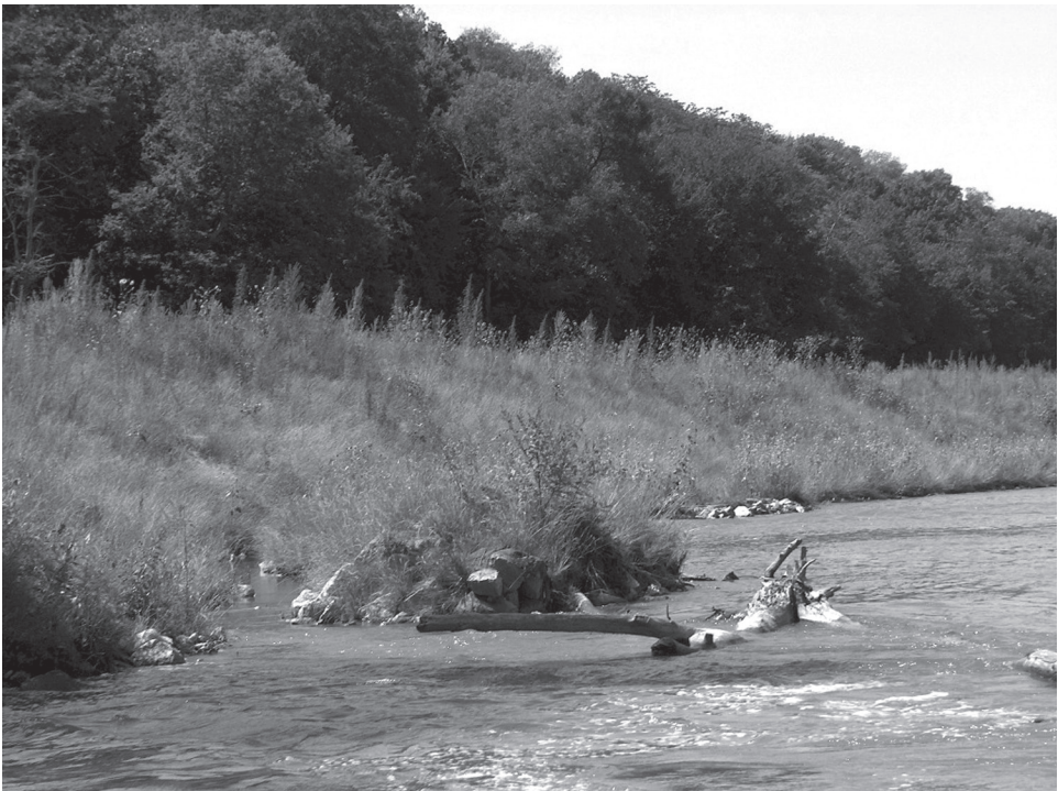
This vegetated bank situated below the forested river bluff is an example of a riverbank stabilization project that has been covered with topsoil and seeded.
