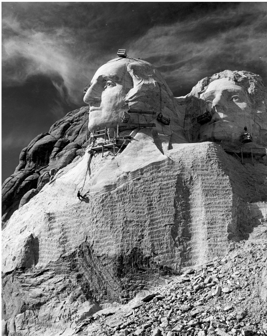
Dangling from their harnesses, workers put the finishing details on the heads of Washington and Jefferson. Image by Verne's Photo.
