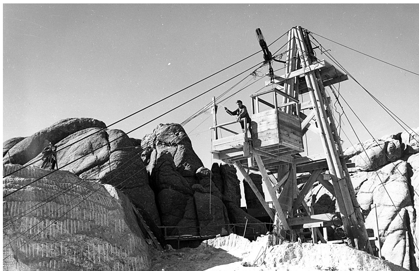
A derrick on top of the mountain and a hoist below kept the bucket going up and down.
