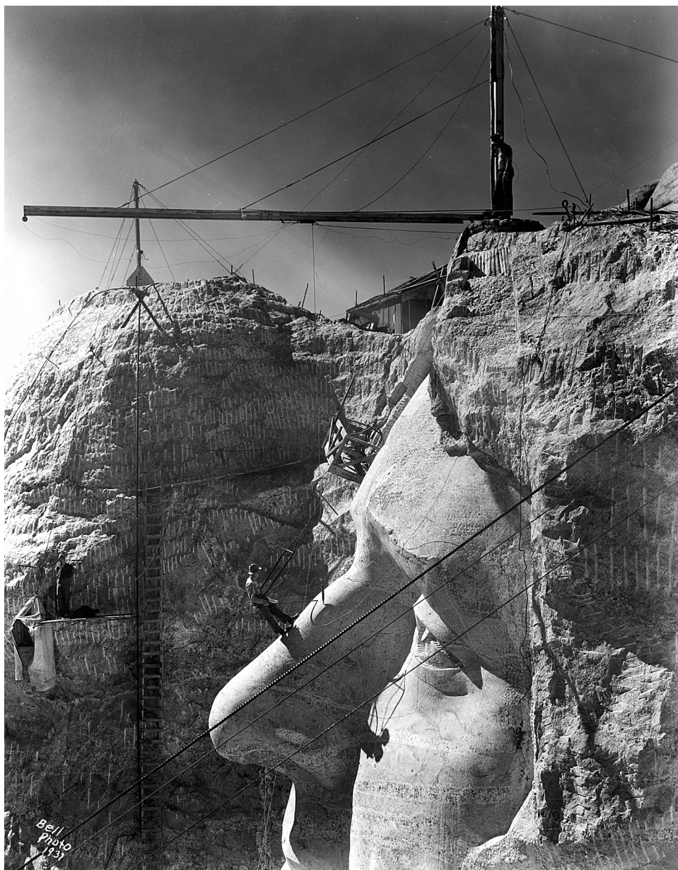
An invention of Gutzon Borglum's allowed workers to transfer measurements from scale models onto the mountain. Image by Bell Photo.
