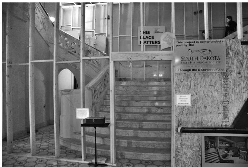
The wooden structure seen here supports the scaffolding used by workers repairing the ceiling plaster near the grand staircase of the Mead Building.
