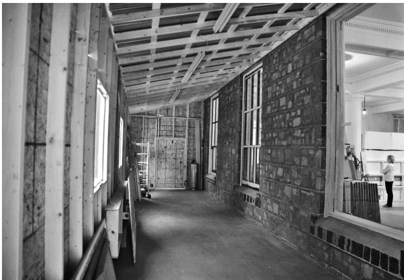
This temporary wooden structure encloses a section of the porch to help ensure a lead-free environment for those working on the window renovation project inside.
