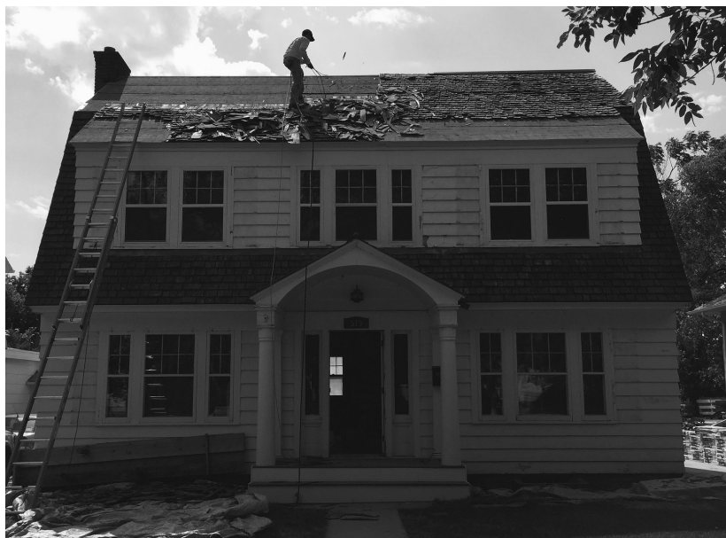
A worker removes old shingles at the start of a project to rehabilitate the Miller House in Pierre.
