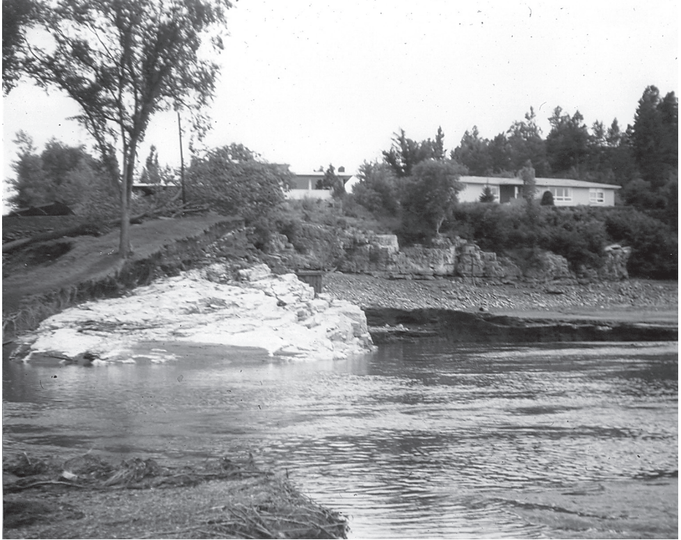
Keith Johnson photographed the damaged Canyon Lake spillway immediately after the flood. The break resulted in a surge of water downstream.
