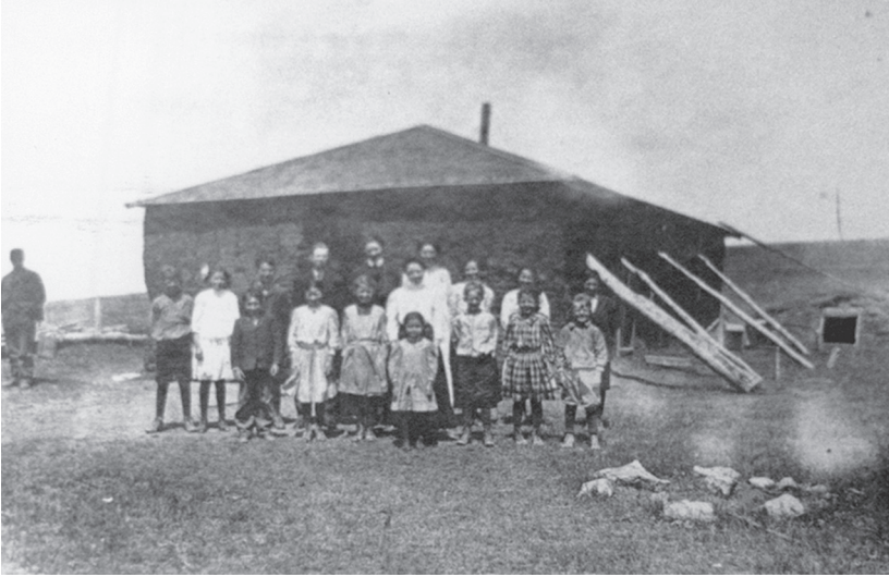
Sagging or bowed walls and the need for bracing plagued many soddies, as seen in this photograph of students gathered in front of their sod schoolhouse.
