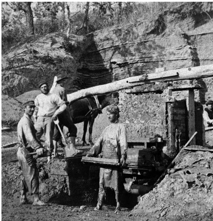
Workers use local materials to make bricks for the construction of permanent buildings at Fort Totten in 1869.
