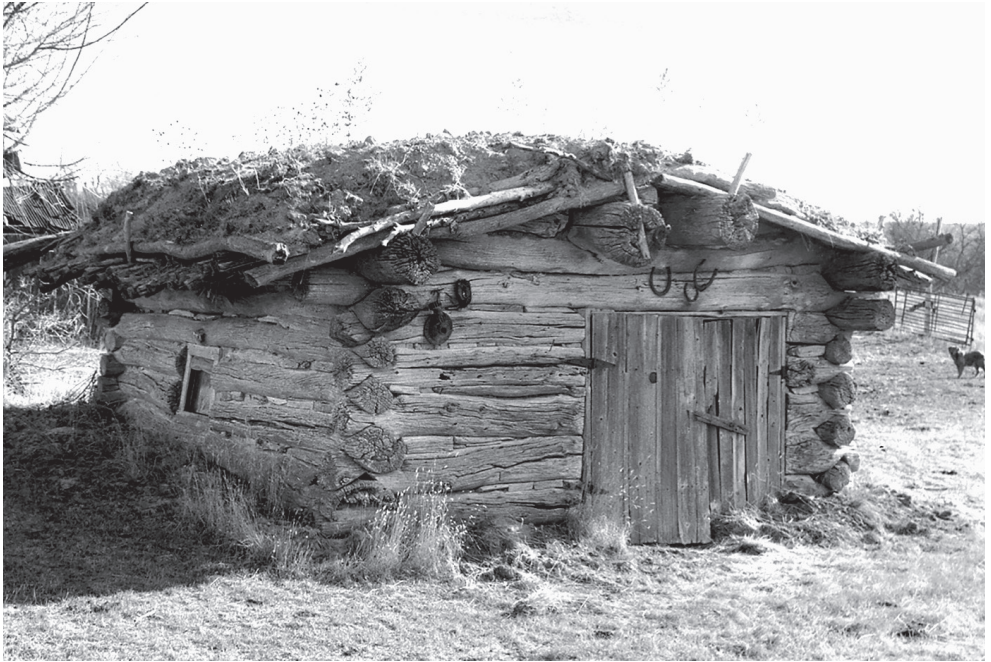
A lack of timber on the prairies and plains restricted the size of log buildings to squat structures, such as the Richards Cabins in Perkins County.
