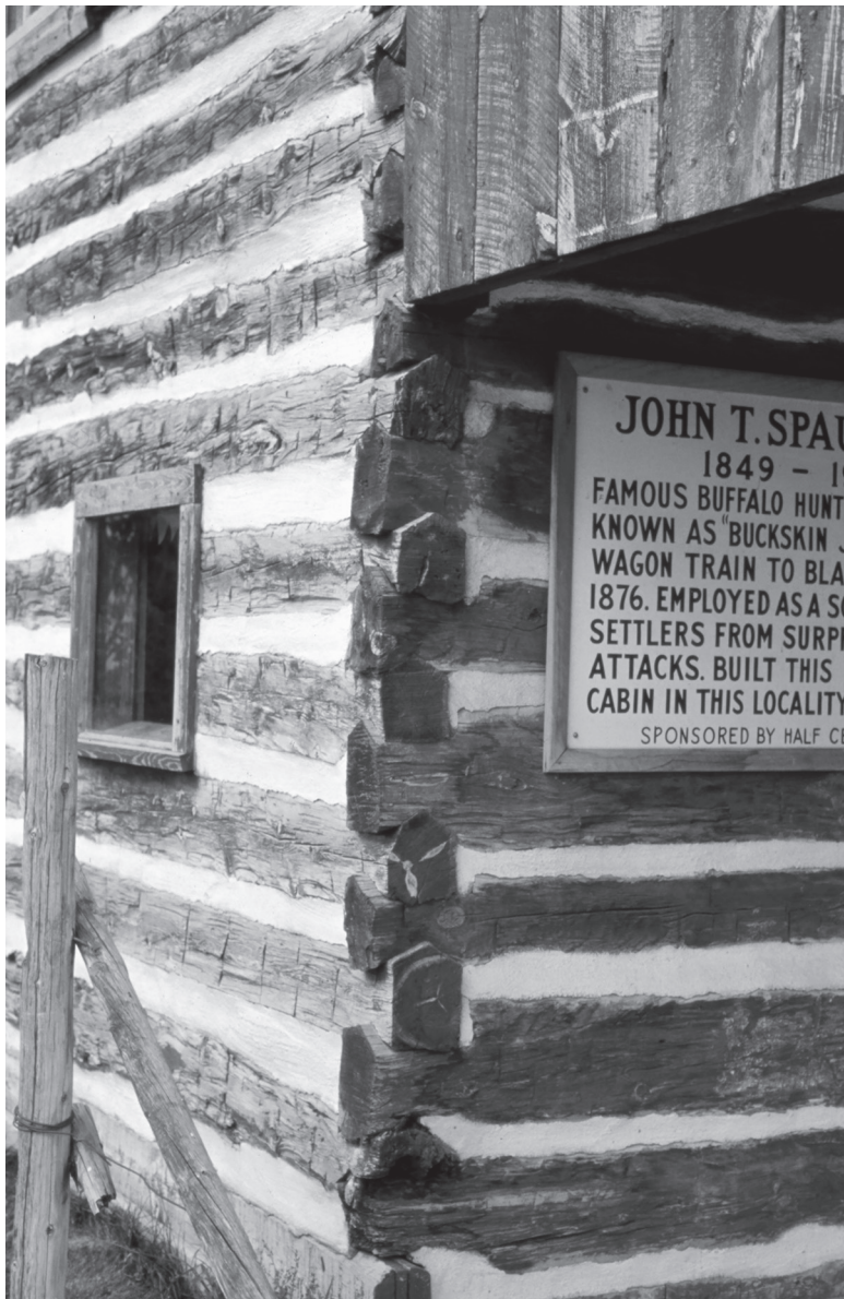
Spaulding’s cabin featured V-notching to connect the walls, a common element among Finnish log constructions as well.
