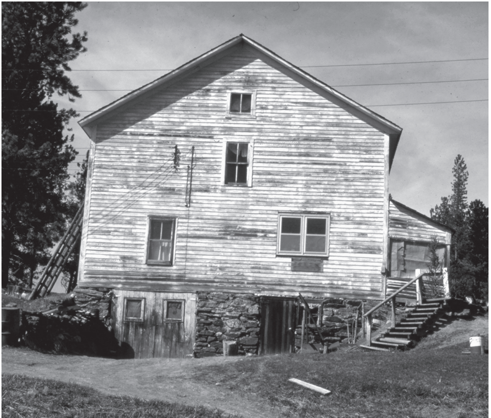
This side view of the main house at the Buskala Ranch shows some of the features common to Finnish log house construction, including exterior ladders (left) and stairways.
