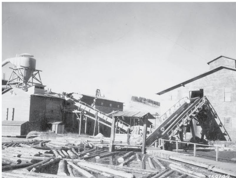
The company's log pond, created by diverting Rapid Creek, allowed it to float logs for easy feeding into the mill via the jack ladder, seen here in 1937.
